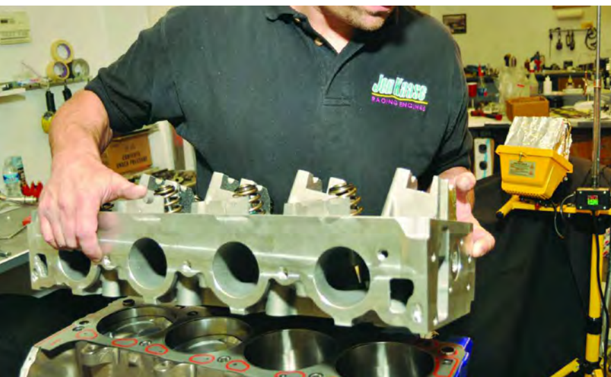
10. Adding heads - Before the cylinder head is installed, silicone sealer is added to both sides and on the ends of the gaskets around the oil drain-back holes. Assembly lube coats the threads and beneath the heads of the 12-point Grade-10 bolts that are torqued to a value of 110lb/ft. Testing has determined that Kaase's Boss Nine heads are worth at least 100hp over the original design.
